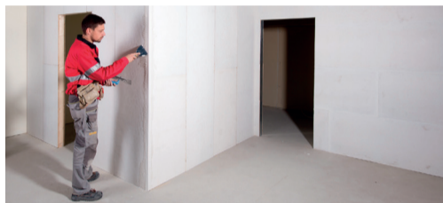
Image 6 Jointing of wall corner
