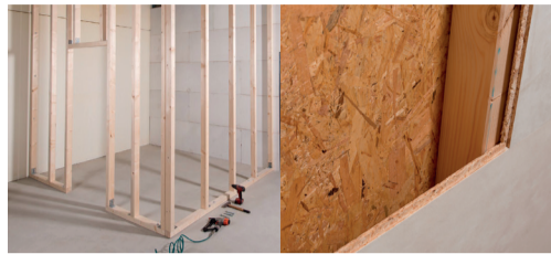
Image 1 Wood frame construction ; installation on wood construction
