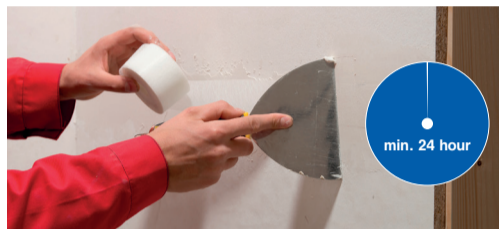
Image 5 Reinforced tape - followed by 24-hour technological break
