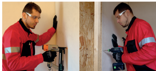
Image 3 Stapling or fastening with screws
