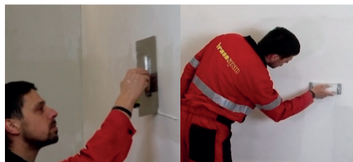
Image 7 Finishing by Firestop finish putty; sanded if necessary
